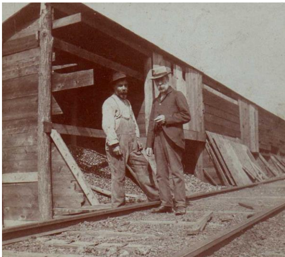
William Schwartz on the left stands by the coal bins along Nye Street
